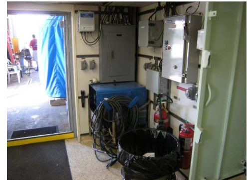
Aft inside corner and doors to staging bay and passage way
